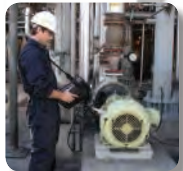
State-of-the-art technology for equipment testing. (ie. Vibration Monitoring & Analysis)
